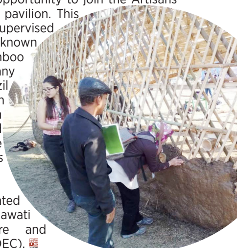
Plastering mud as organic cement on the bamboo pavilion.
