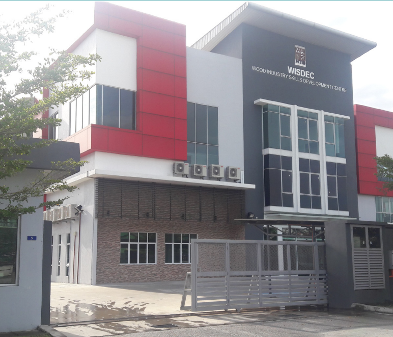
New building for training centre known as WISDEC 2
