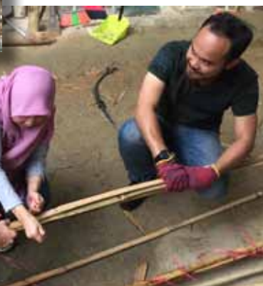
Making rafters for roofing.
