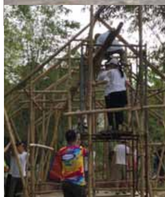
The construction of Organic Bamboo Sala.
