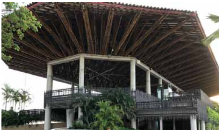
Application of bamboo roof truss at the club house in Bogota.
